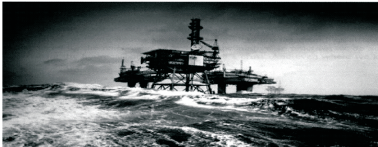
Figure 55: Offshore Production Platform
