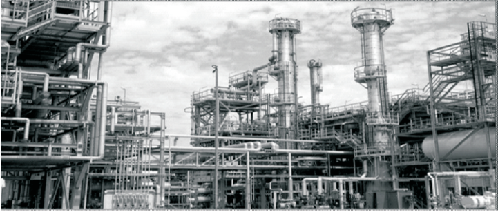
Plate 9: The Port Harcourt Refinery
