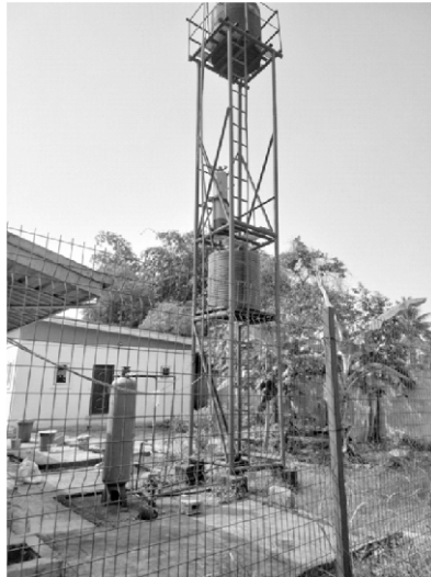
Plate 1: A typical packed bed water treatment unit for a household at Unyengala, Andoni
