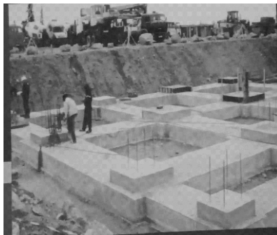
PLATE: 5. Construction of a high rise building with basement..
