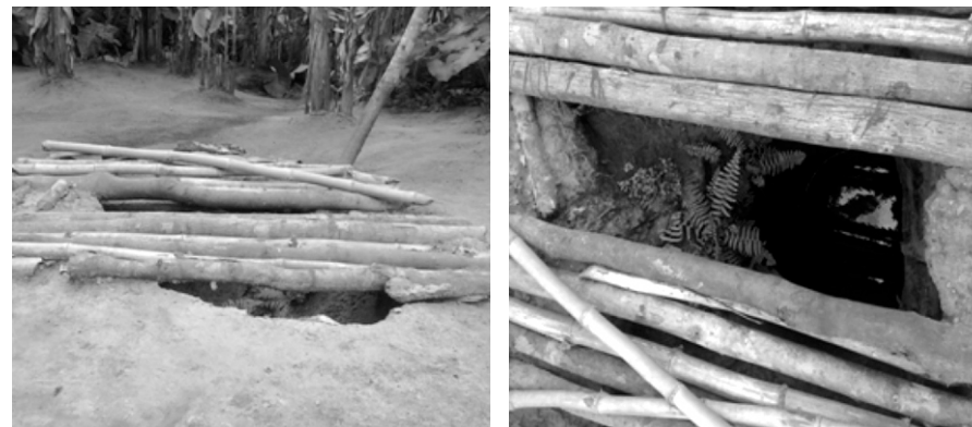
Plate 5e: Location D - Well in Amalem community collapsed after rains (Obire and Alali, 2015)
